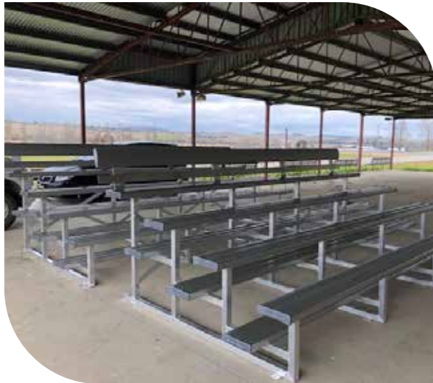
With the grandstands built, we are just waiting on new signage to be completed!
